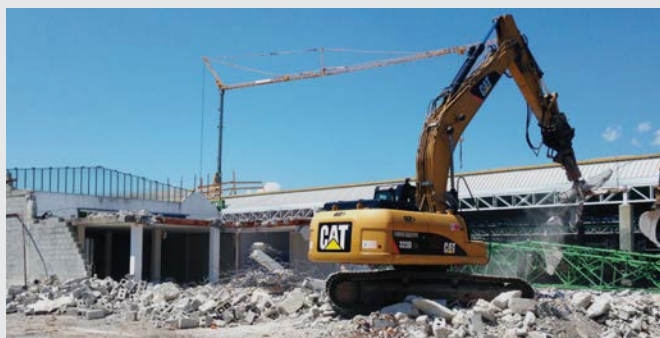
Demolition of old premises
