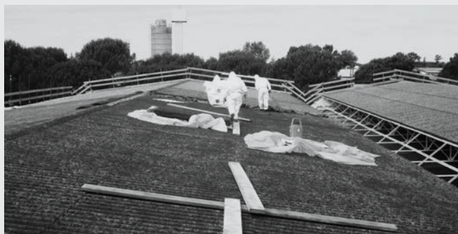
Asbestos removal
